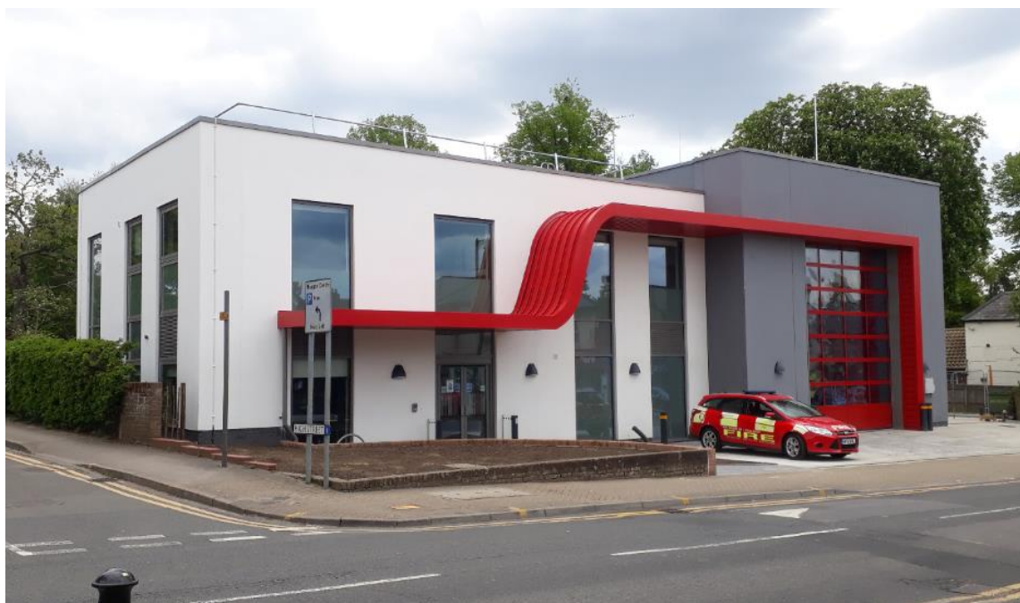
Figure 5 – Crowthorne Tri-Service Community Station (completed 2020).
